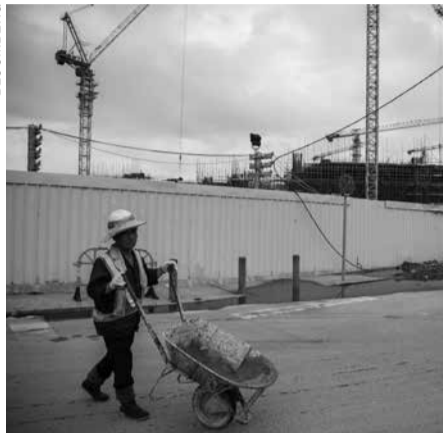
A worker pushes a cart in front of the construction site of the Lisboa Palace
