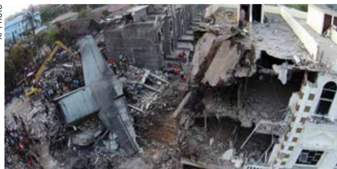
The site where an Indonesian air force cargo plane crashed in Medan
