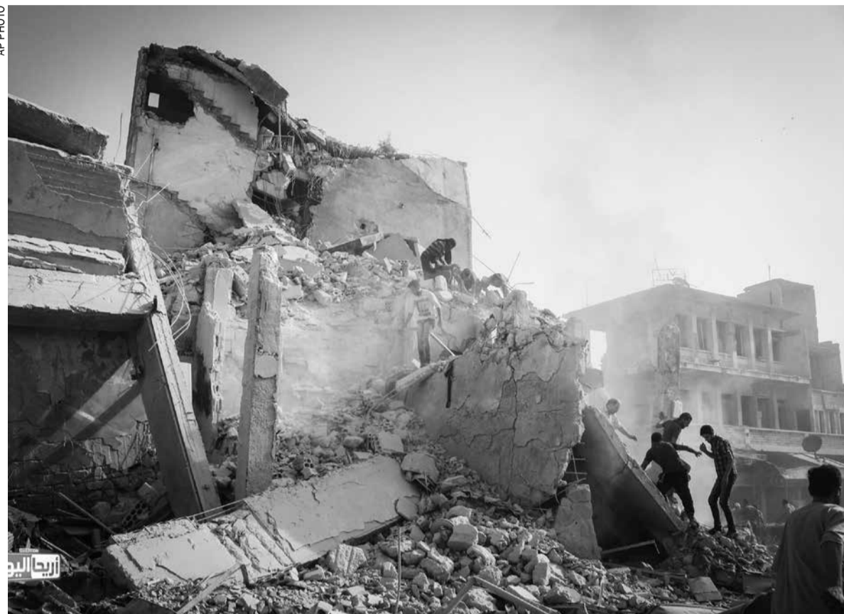
Syrian citizens look for survivors under the wreckage of a destroyed building that was damaged after a government warplane crashed in the center of the town of Ariha, in the northwestern province of Idlib
