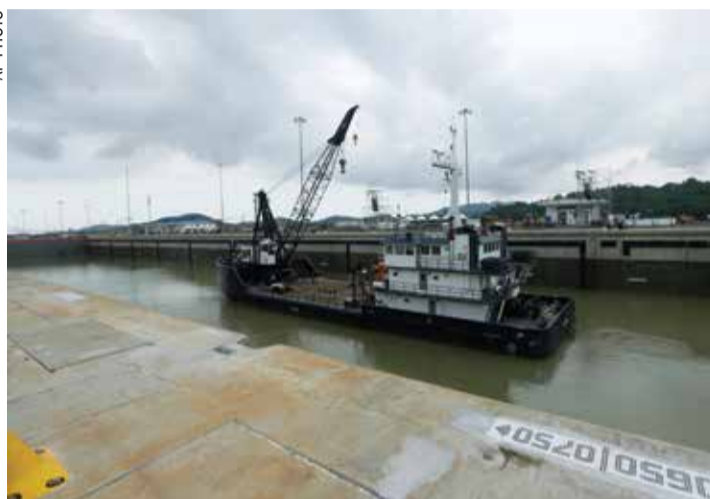
Panama Canal Authority crane ship Oceanus, navigates the Cocoli locks during a test of the newly expanded Panama Canal locks on Pacific side
