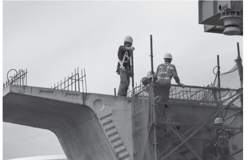
LRT construction works
