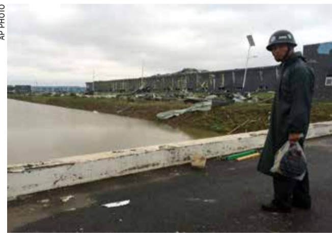
A policeman stands near a damaged building in Funing county in Yancheng city in eastern China's Jiangsu Province
