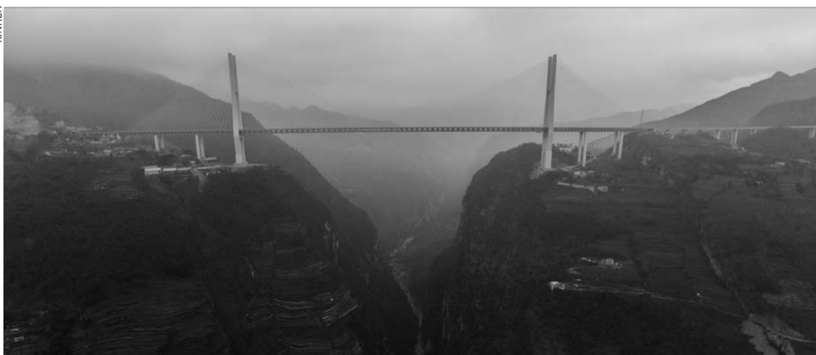
The Beipanjiang Bridge, in southwest China's Guizhou Province, was inaugurated yesterday. The 1341.4-metre-long bridge soars 565 metres above a river and is considered the world's highest bridge
