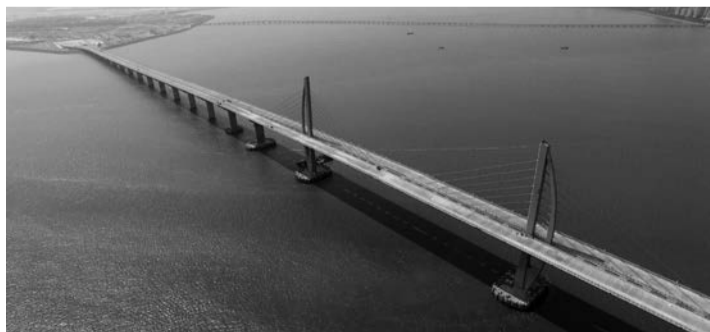
The Hong Kong-Zhuhai-Macau bridge
