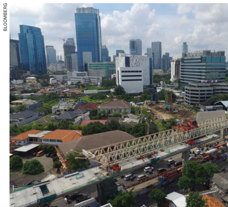
A highway stands under construction in Jakarta
