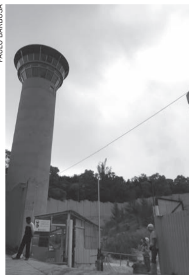
The Ka Ho prison is currently under construction
