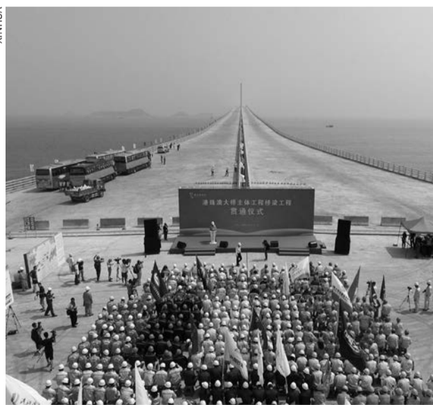
The HK-Zhuhai-Macau bridge is nearing completion
