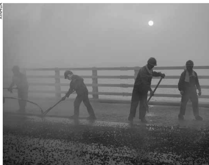
Builders use asphalt to surface the Hong Kong-Zhuhai-Macau Bridge
