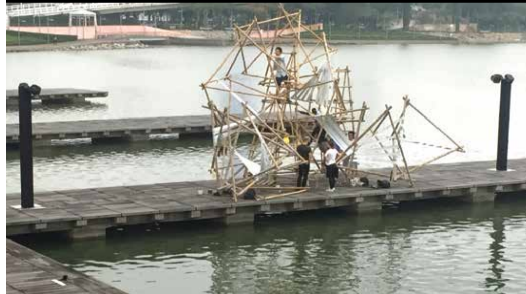
University of Saint Joseph third-year undergraduate architecture students set up a temporary structure besides the Sai Van Lake. The Elapse Pavilion will be inaugurated today. The structure is made of bamboo poles, steel-rod connections, and nylon ropes.
