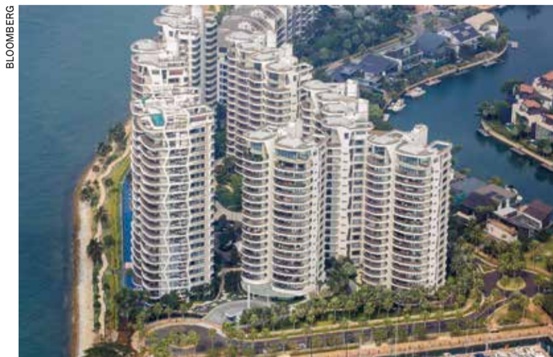
Residential buildings in Singapore
