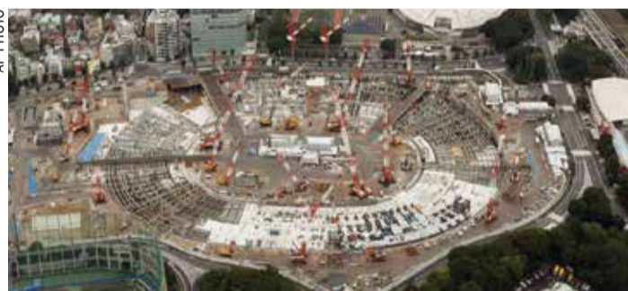
Japan's new National Stadium is seen under construction in Tokyo
