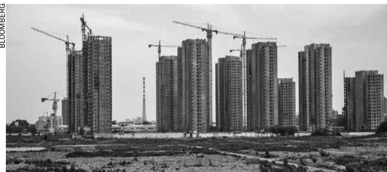
Residential buildings stand under construction in Jining, China
