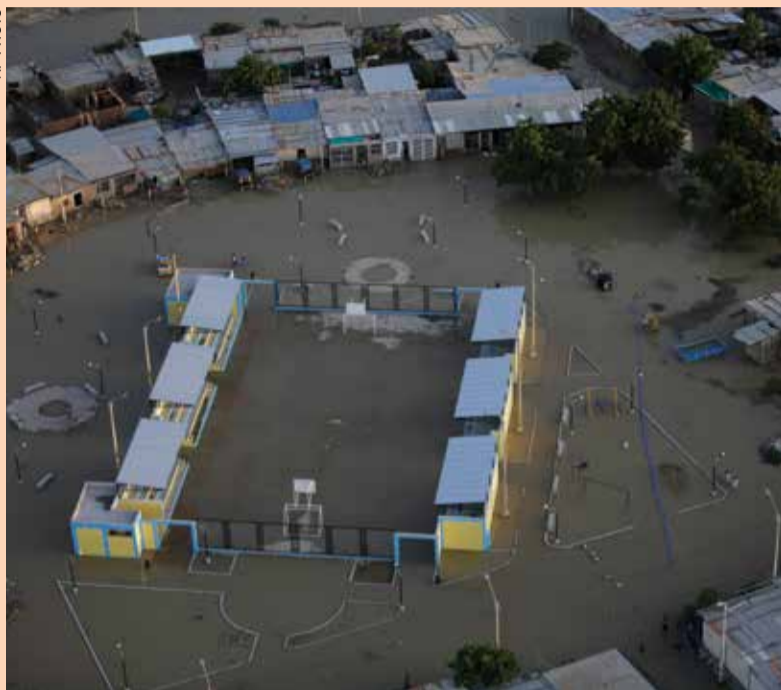
A flooded neighborhood is seen from the air in Piura
