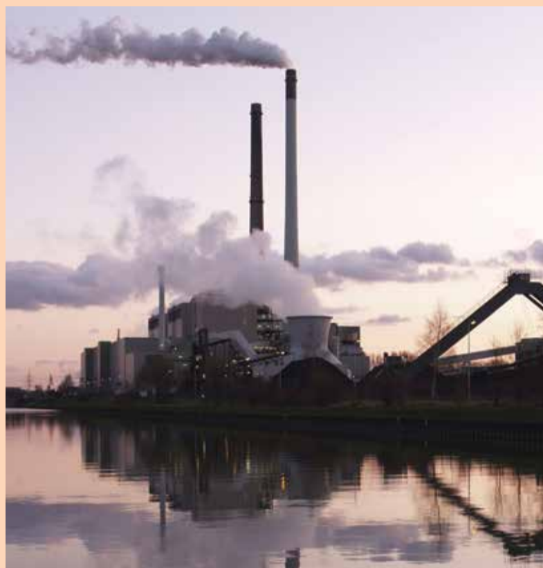
A coal power plant
