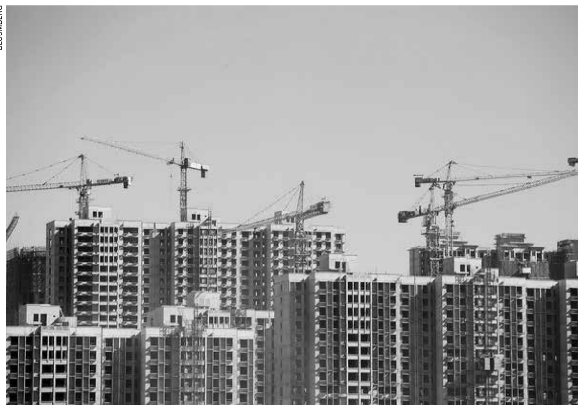
Cranes operate at a residential construction site in Beijing
