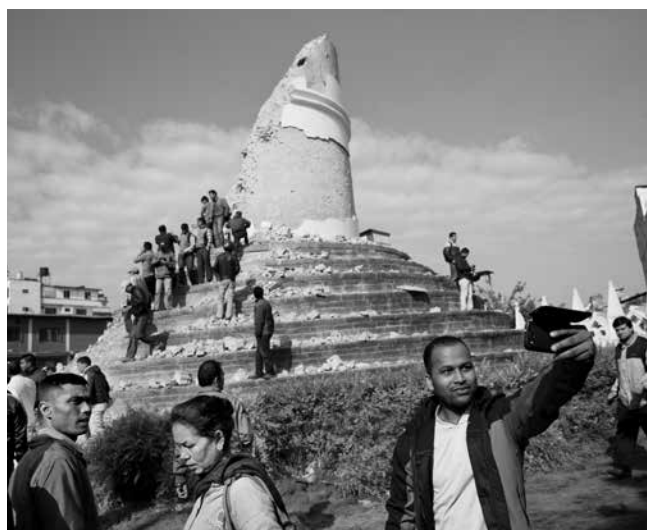
A man takes a selfie at the historic Dharahara Tower, a city landmark that was damaged in the quake
