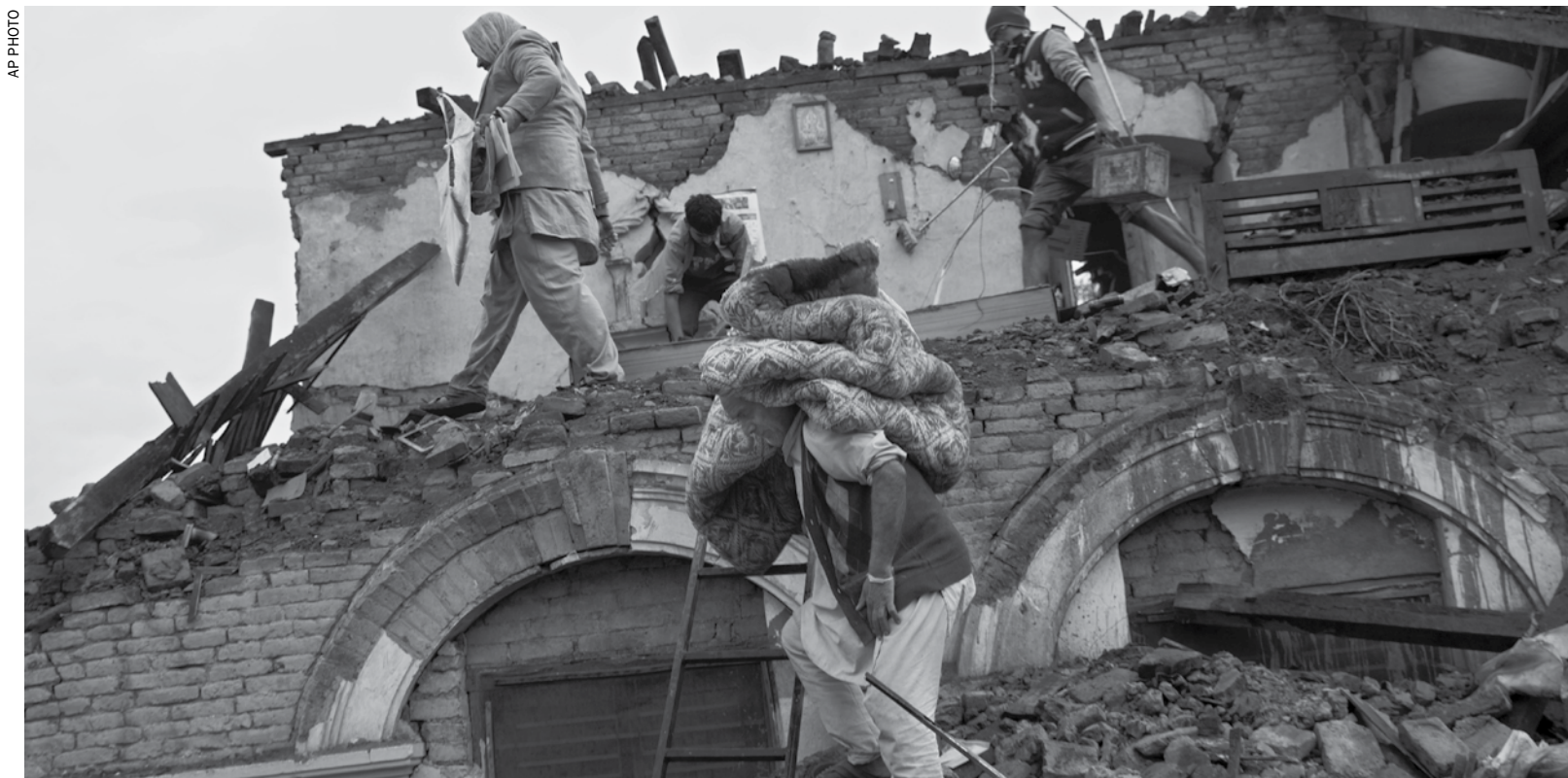
Residents rescue items from debris of a house that was damaged in Saturday's earthquake in Kathmandu
