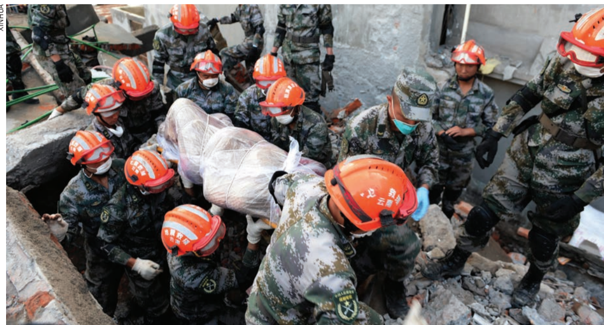
Chinese rescuers carry the body of a victim at a building collapse site on the outskirts of Kathmandu, Nepal
