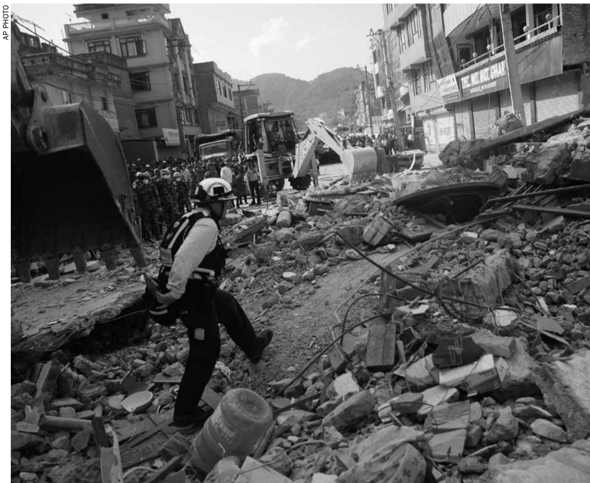
A rescue worker from USAID inspects the site of a building that collapsed in an earthquake in Kathmandu
