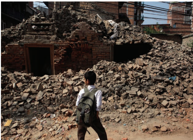
A Nepalese boy walks past a collapsed building close to his school in Kathmandu
