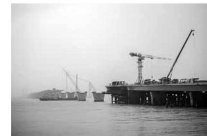
The Hong-Kong-Zhuhai-Macau bridge
