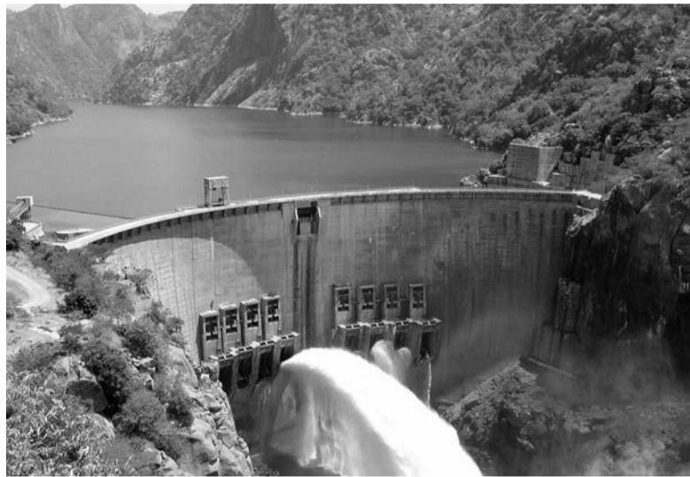
Cahora Bassa Hydroelectric Dam
