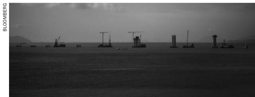
Cranes operate on the Hong Kong-Zhuhai-Macau bridge currently under construction
