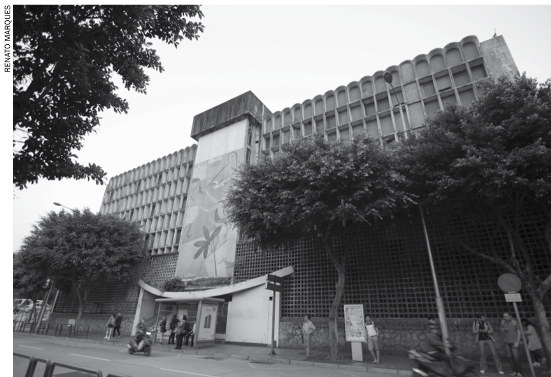
Hotel Estoril's façade
