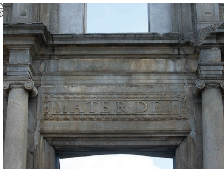
The St. Paul's Church façade, built in 1602-1640, is one of the elements analyzed in the documentary to be aired by National Geographic
