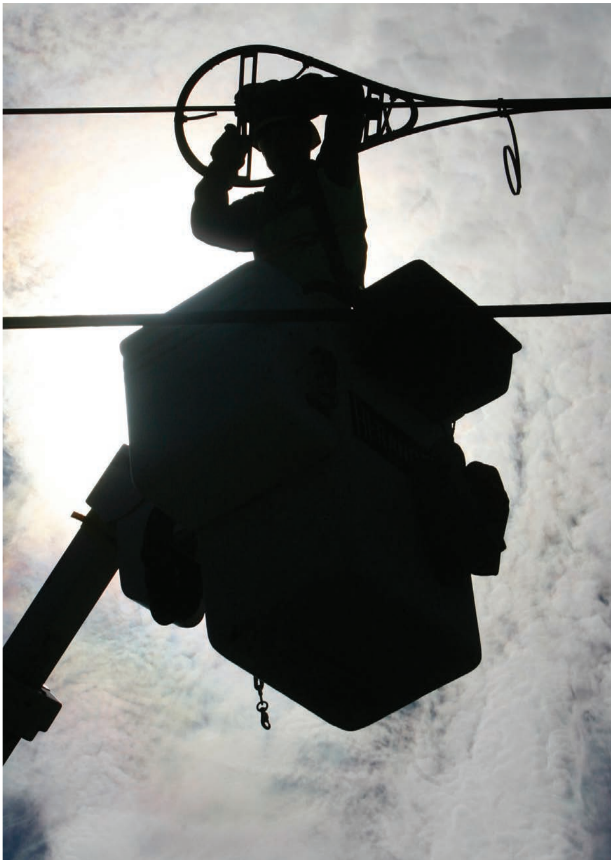
A.J. Bowen works on fiber-optic installation in Norton, Vt.
