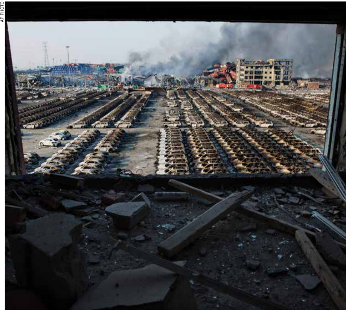
A shattered window frames the site of the explosion at the port warehouse in northeastern China's Tianjin municipality
