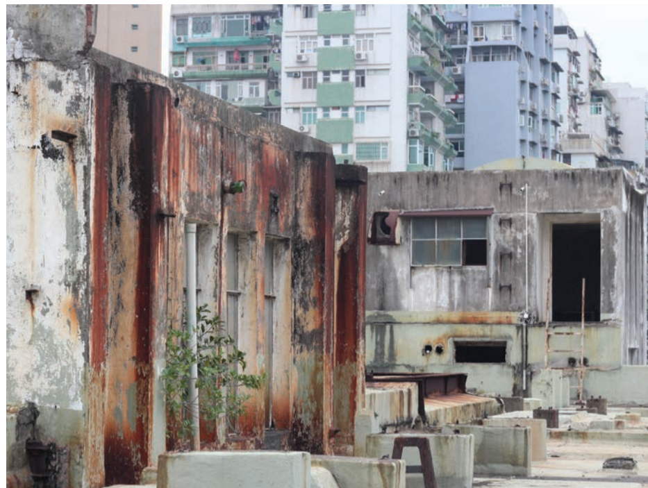
A view of the rooftop
