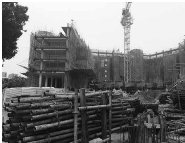
Construction works on USJ's new campus
