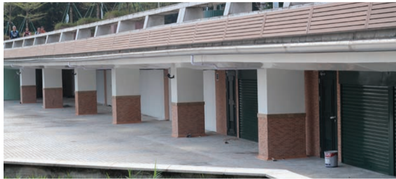
Aspect of the area after the renovation works conducted by IACM
