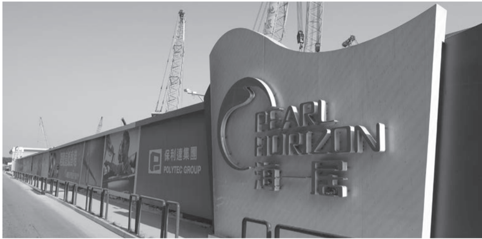
The Pearl Horizon construction site
