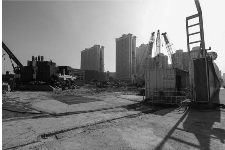
The Pearl Horizon construction site
