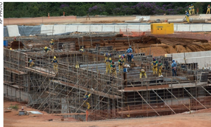
Construction workers build Deodoro Olympic Park in Rio de Janeiro
