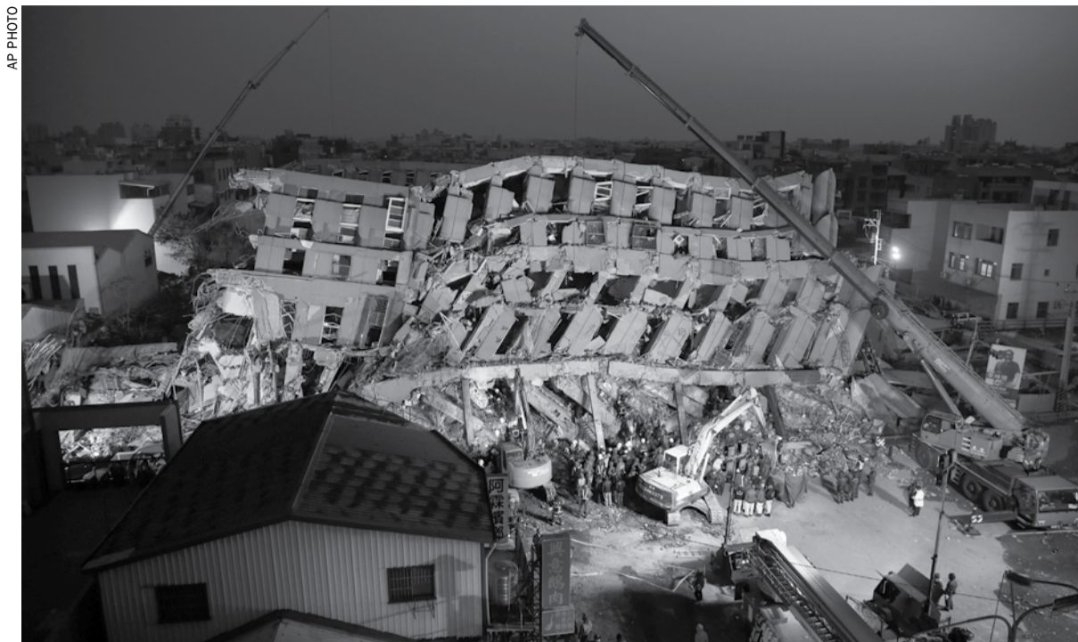
In the early morning, emergency rescuers continue to search for the missing in a collapsed building from an earthquake in Tainan
