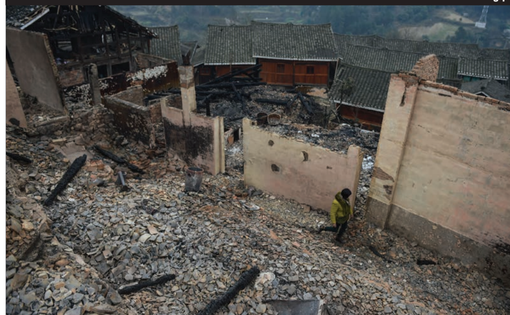
A villager walks beside a damaged house after a fire in Wenquan Village, located at southwest China's Guizhou Province. A fire broke out Saturday evening in the village, affecting 120 people and damaging more than 60 houses.
