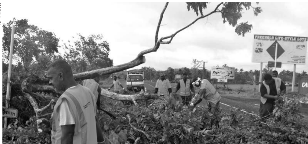
Road workers remove a fallen tree blocking a road near Lami
