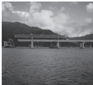
The under construction Hong Kong-Zhuhai-Macau Bridge
