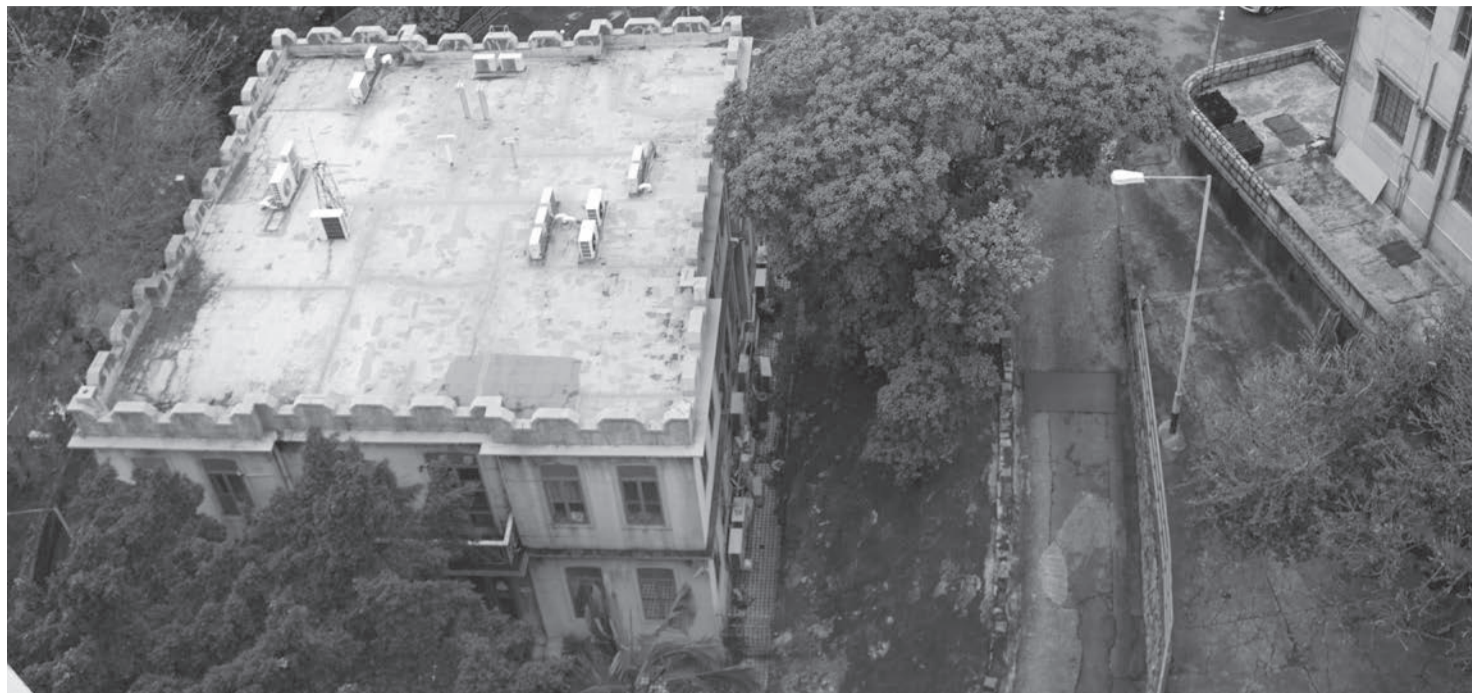
The two buildings beside the public hospital planned for demolition
