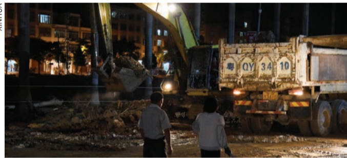
An excavator works to clear silts in Xinyi, Guangdong Province
