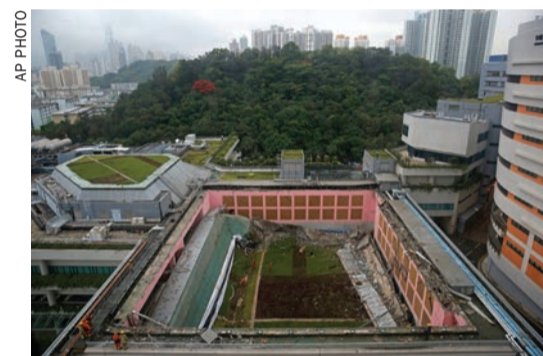
An aerial view shows firefighters walking on the debris of the collapsed section of a building at the City University's campus
