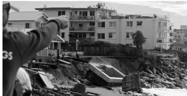
A swimming pool is dislodged and lays on a beach after storms undermined the pilings at Collaroy in Sydney
