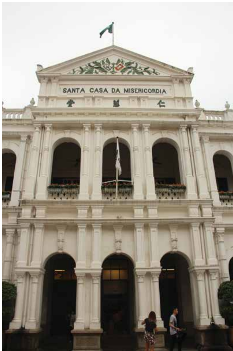
The historical Holy House of Mercy building
