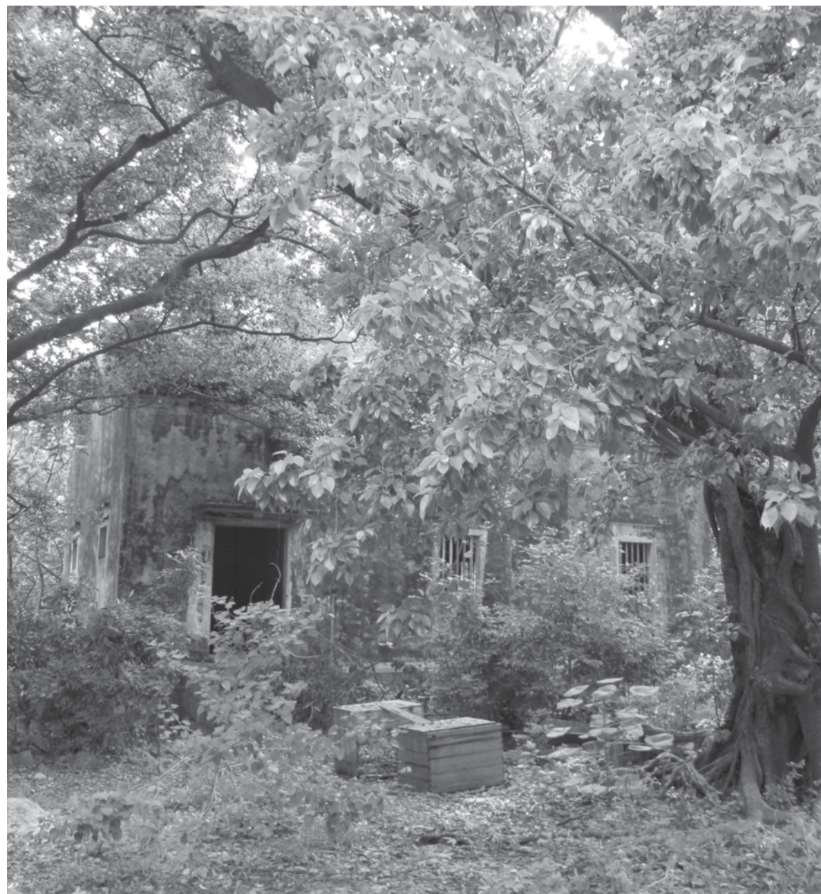
Aspect of the old factory and surrounding area
