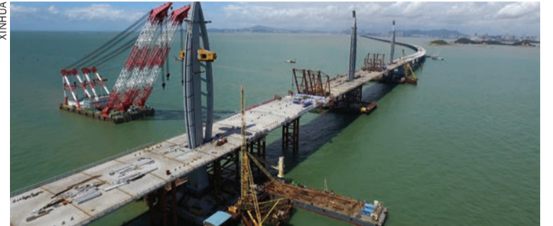
Construction works on the Hong Kong-Zhuhai-Macau bridge
