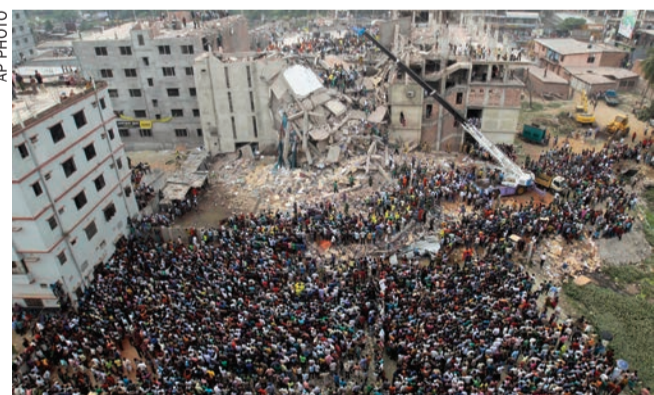
In this April 2013 photo, Bangladeshi people gather as rescuers look for survivors and victims at the site of a building that collapsed in Savar, near Dhaka
