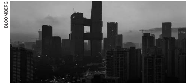
A view of Tencent's future headquarters, still under construction, in Shenzhen
