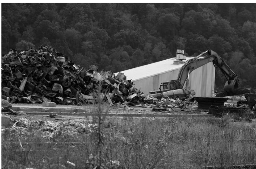
The area that housed the dry scrubber
