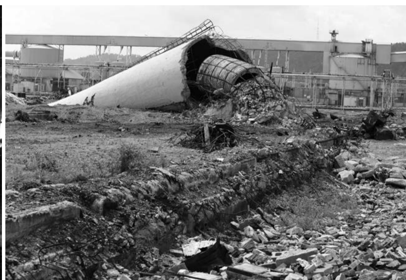
One of the stacks from the furnace room
