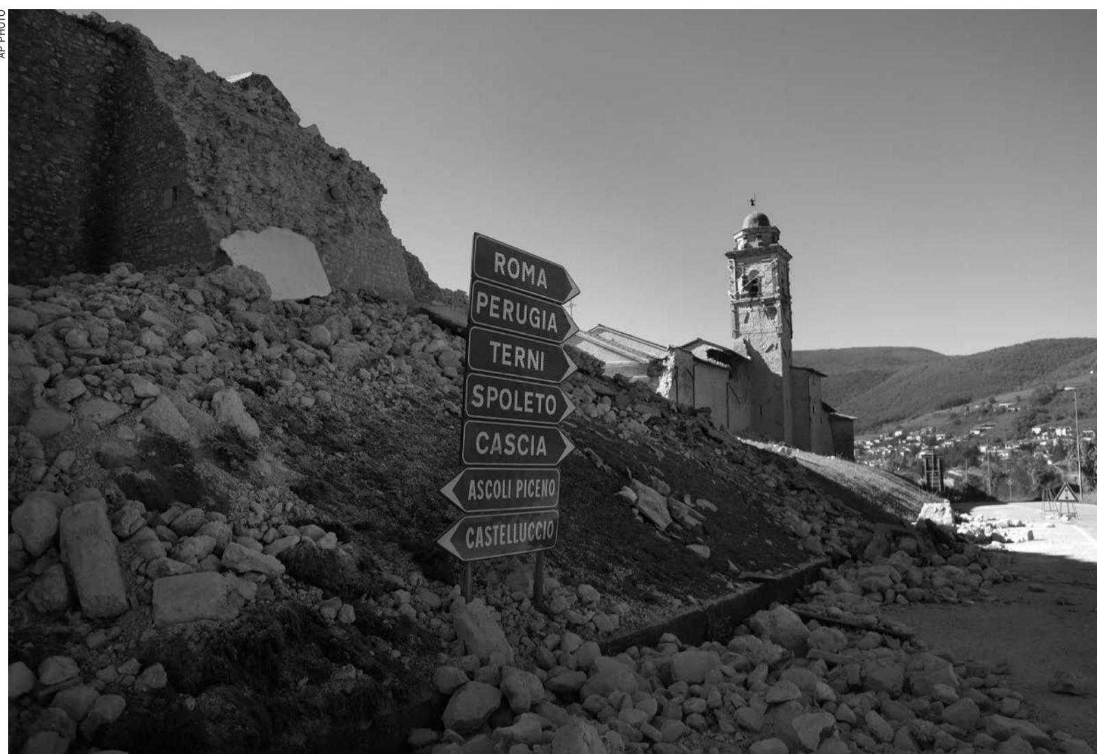
The tower of the Church of the Madonna of the Angels is still standing amidst rubble on a road near Norcia
