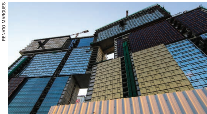
The MGM Cotai construction site pictured in February 2016
