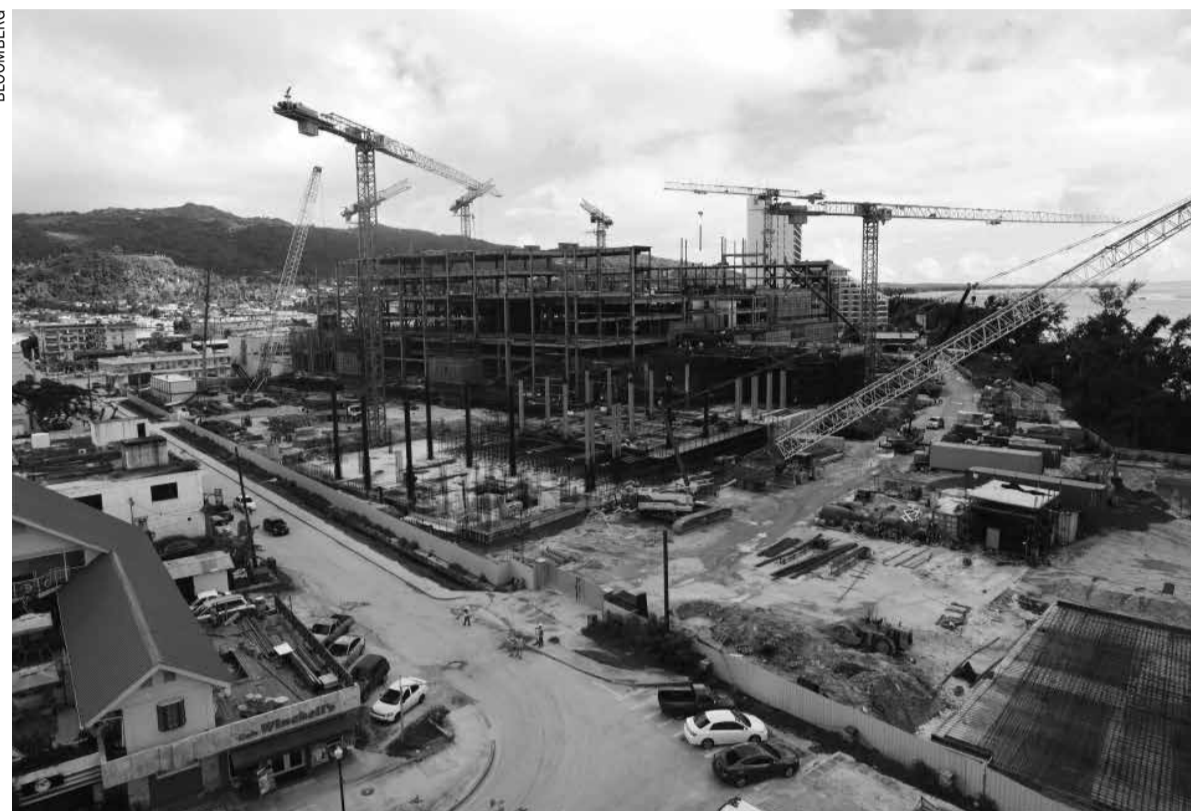
The construction site of the new resort
