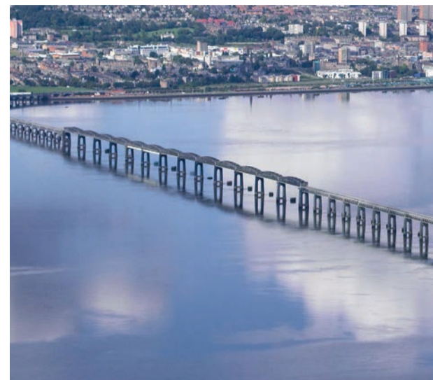
The bridge as it looks today
